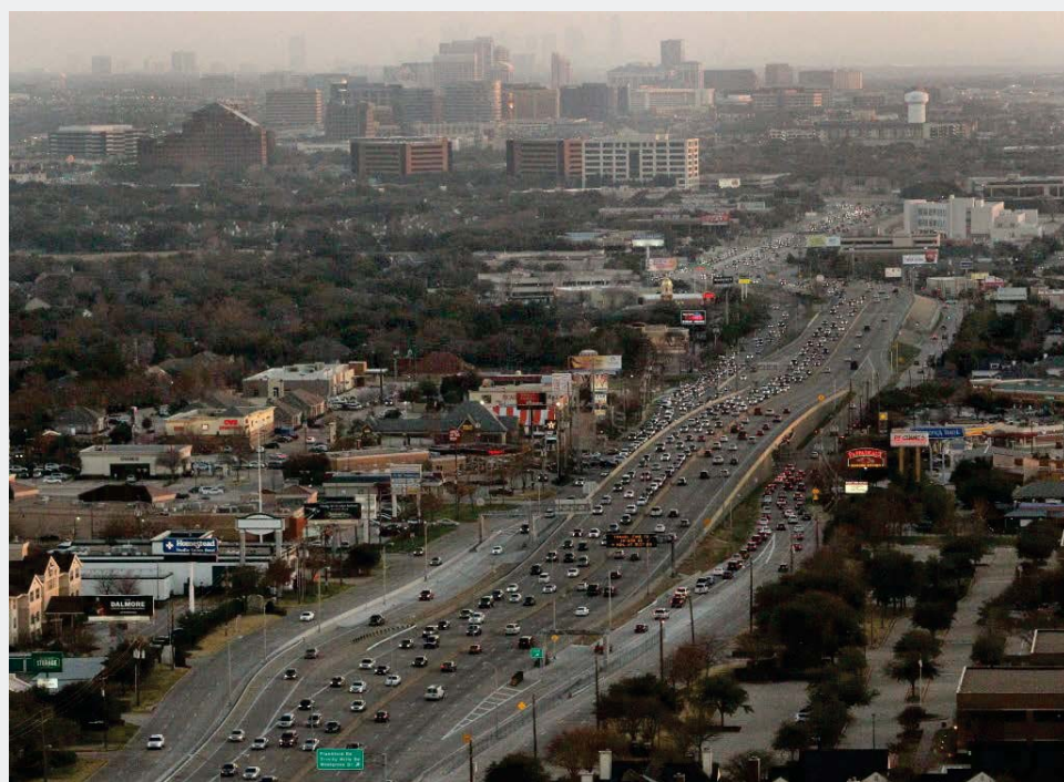
What if the problem with our commutes is not just that they take too long, but they are too long in the first place? Even billions in tolled infrastructure, such as the DNT above, can't keep the cars moving freely in a fast-growing area like North Texas. (Louis DeLuca / Staff Photographer)
