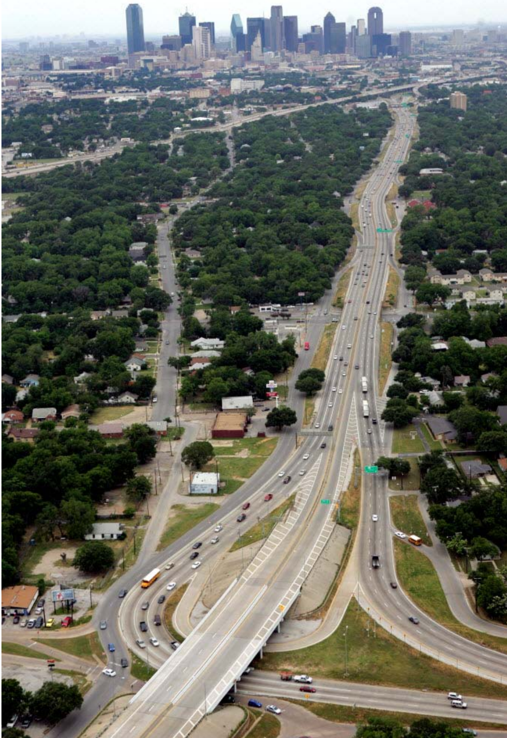
The primary aim of the S.M. Wright Boulevard project has always been to eliminate "Dead Man's Corner" on US 175, where C.F. Hawn Freeway (bottom, far right) curves sharply to become S.M. Wright Freeway (vertical line going north towards Dallas). The construction of S.M. Wright divided a community, and residents today hope that plans to downsize the freeway will include plans for revitalization as well. Photographed May 13, 2010.
